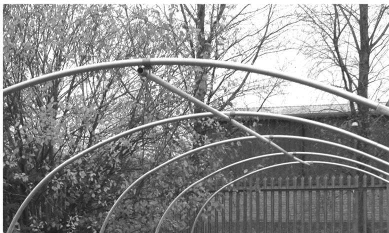
Completed centre ridge.
