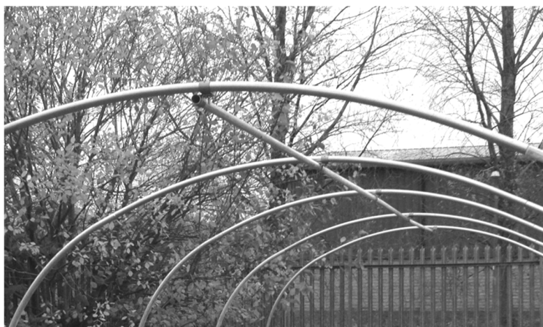
Completed centre ridge.
