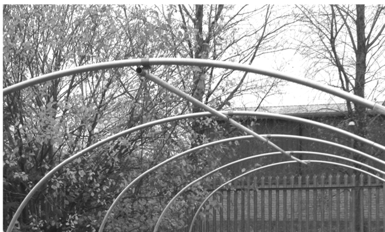
Completed centre ridge.
