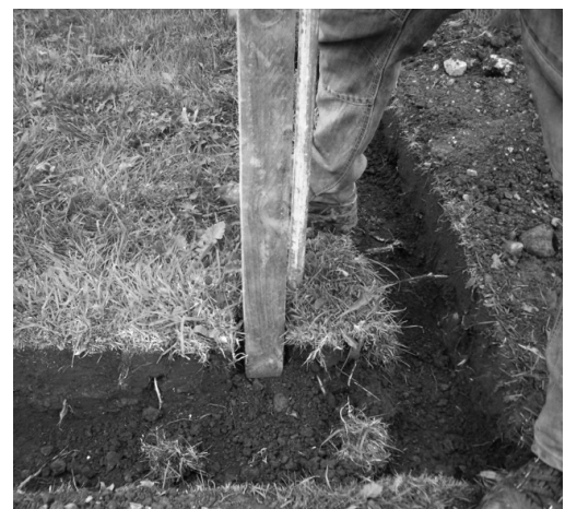
Fig109 – vertical positioned in trench/dug out
