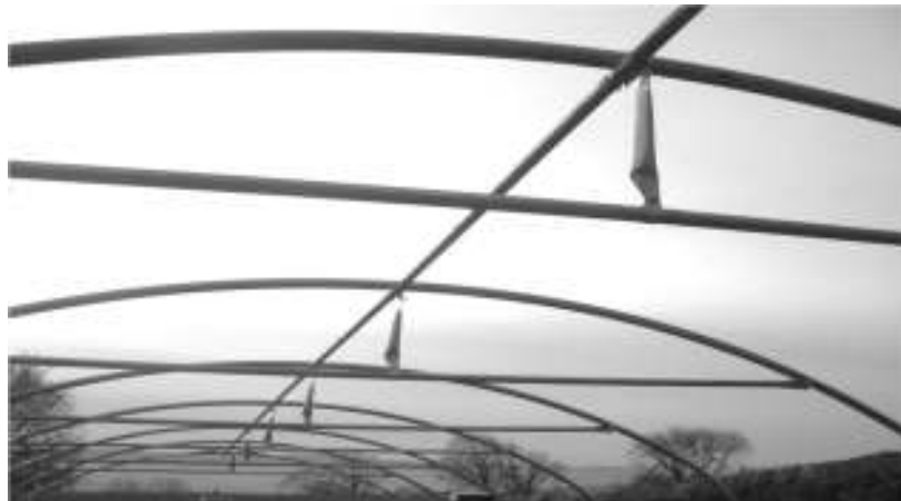
Completed crop bars and supports fixed to all intermediate hoops
