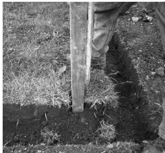
Fig90 – vertical positioned in trench/dug out
