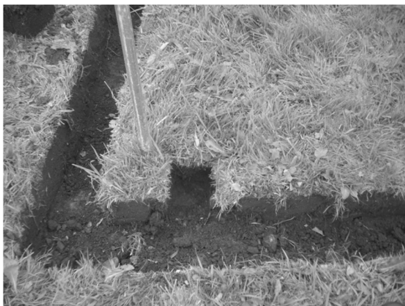
Fig89 – ground dug out for vertical
