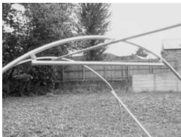
Completed Centre Ridge.
