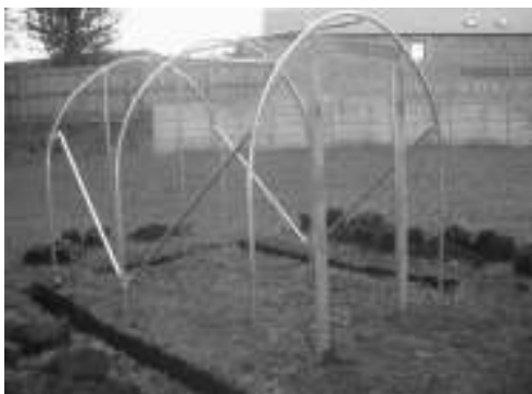
Fig50 – Starting to dig the trench
