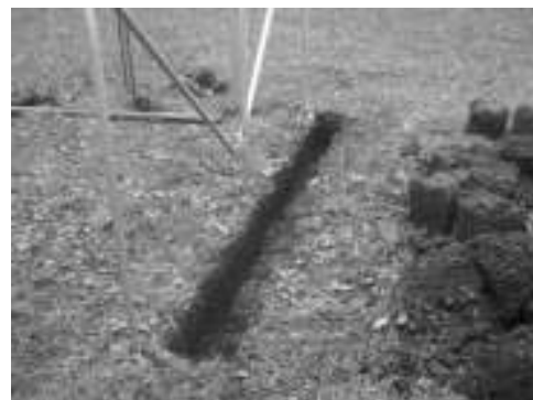
Fig51 – Starting to dig the trench
