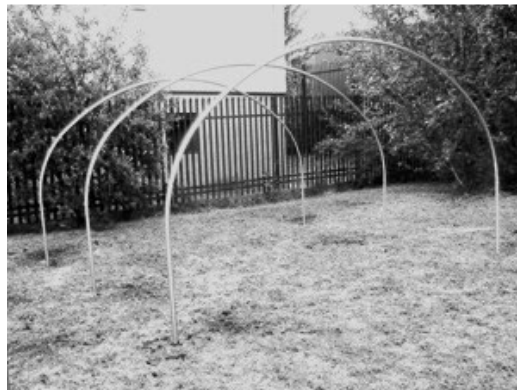
Fig10 – Hoops in position on Foundation Tubes.
