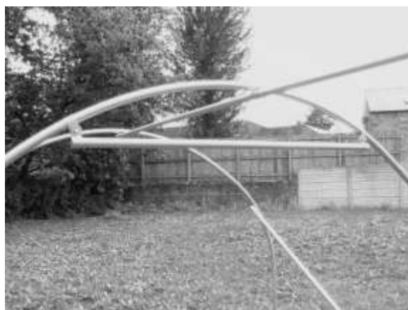
Completed Centre Ridge.
