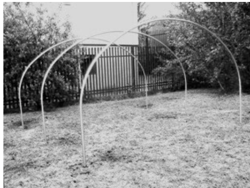
Fig10 – Hoops in position on Foundation Tubes.
