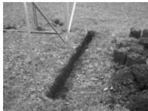
Fig35 – Starting to dig the trench
