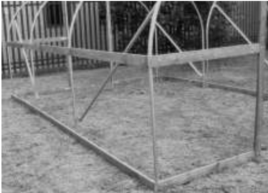
Fig44 – Base Rail at ground level. Side Rail at top of straight side.
