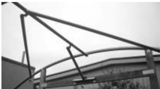
Fig14 – Roof Stabilisers before fitting cover.
