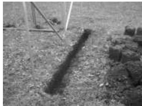
Fig32 – Starting to dig the trench
