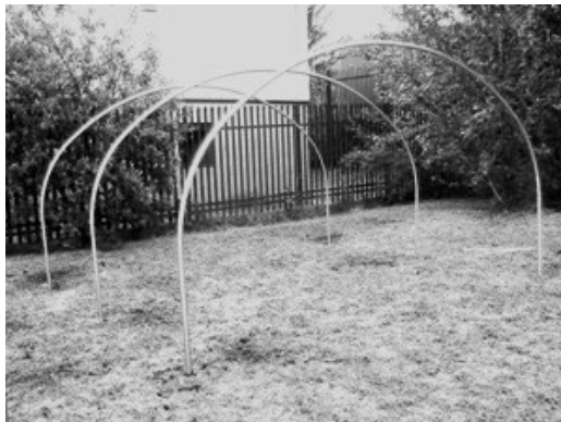
Fig10 – Hoops in position on Foundation Tubes.
