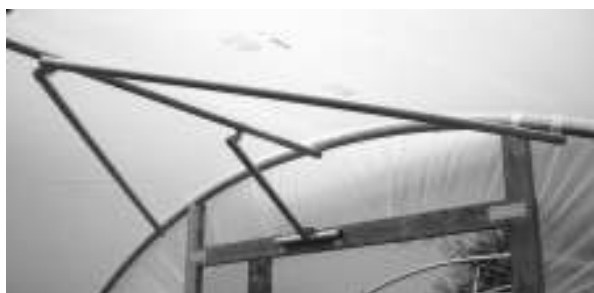
Fig15 – Roof Stabilisers after fitting cover.
