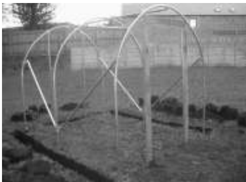
Fig31 – Starting to dig the trench
