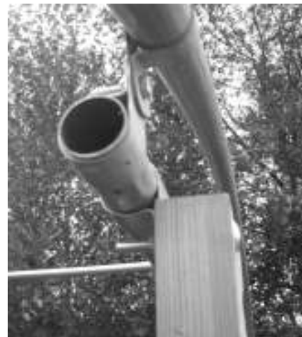
Fig16 – Showing Door Rail inline with the inside edge of the end hoop.
