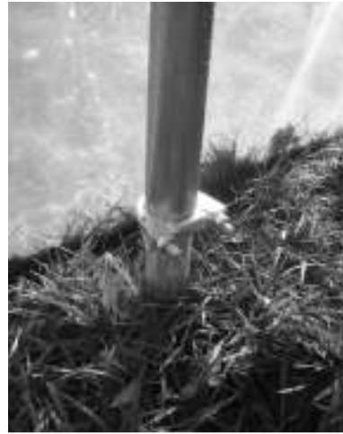
Hoop raised and clamped in position over the foundation tube (with hoop sitting on clamp)
