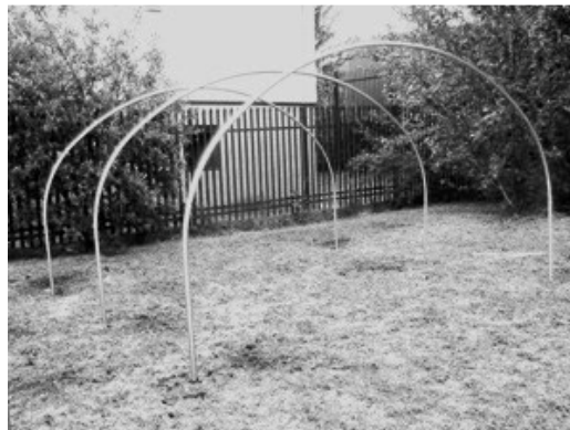
Fig10 – Hoops in position on Foundation Tubes.
