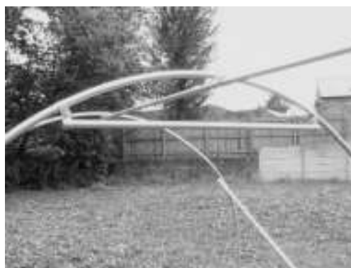
Completed Centre Ridge.
