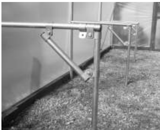
Completed Staging Supports, with loose P Clip for fixing your own timber top.
