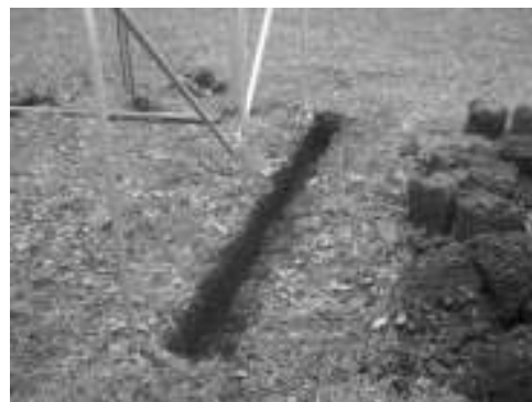
Fig55 – Starting to dig the trench
