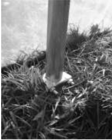
Hoop and clamp slotted over the foundation tube to ground level
