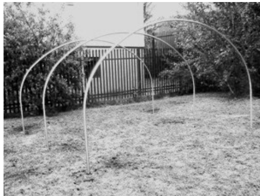
Fig10 – Hoops in position on Foundation Tubes.
