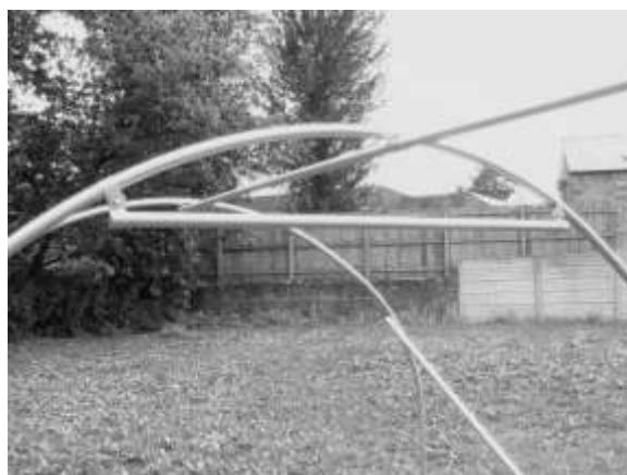
Completed Centre Ridge.
