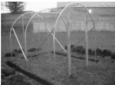
Fig54 – Starting to dig the trench
