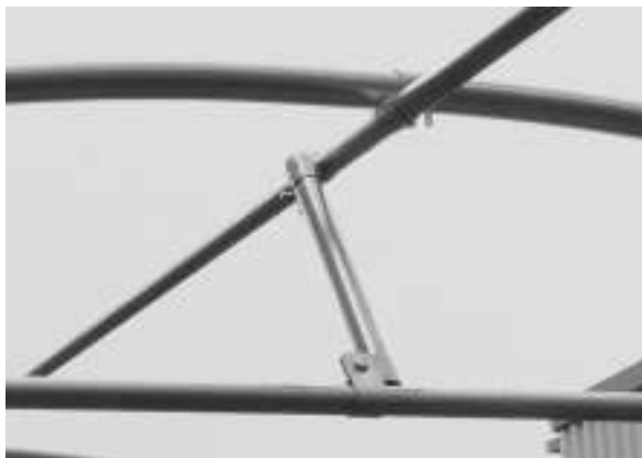
Fig15 – Diagonal support
