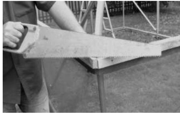
Remove the sharp corner by cutting at an angle.
