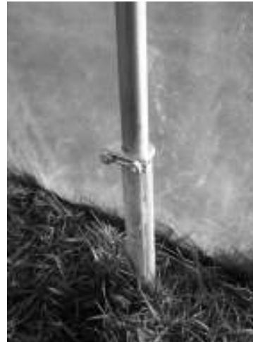
Clamping the hoop into position at the top of the foundation tube.
