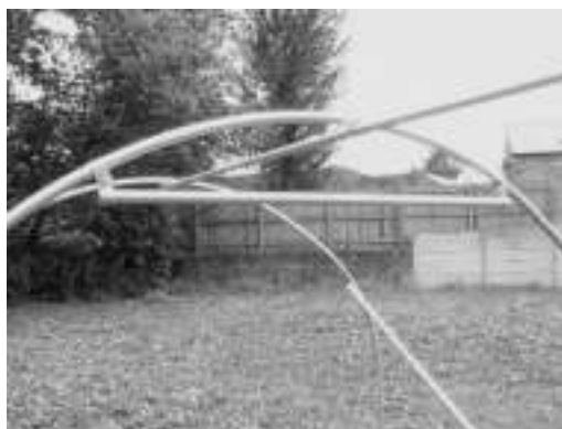
Completed Centre Ridge.
