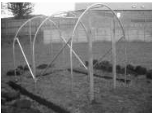
Fig52 – Starting to dig the trench
