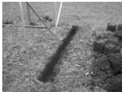
Fig53 – Starting to dig the trench
