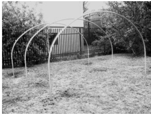
Fig10 – Hoops in position on Foundation Tubes.
