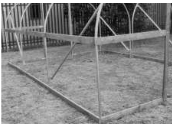
Fig63 – Base Rail at ground level. Side Rail at top of straight side.
