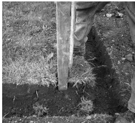
Fig77 – vertical positioned in trench/dug out
