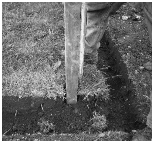
Fig96 – vertical positioned in trench/dug out
